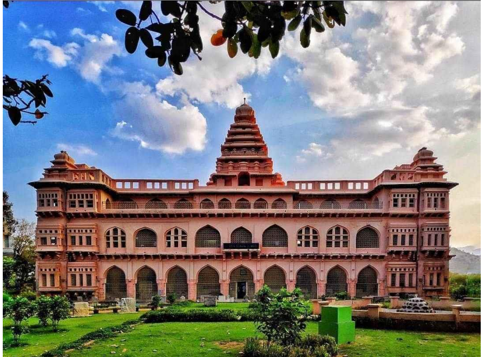
Chandragiri Fort, Chandragiri
